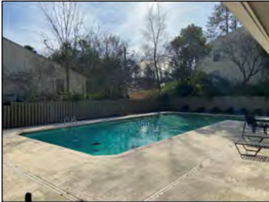
Typical View of Subject Pool
