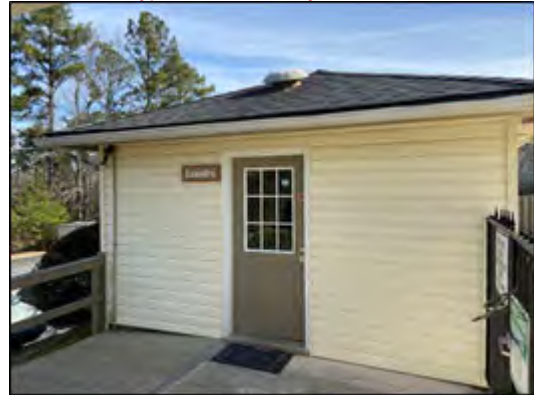
Typical View of Subject Laundry
