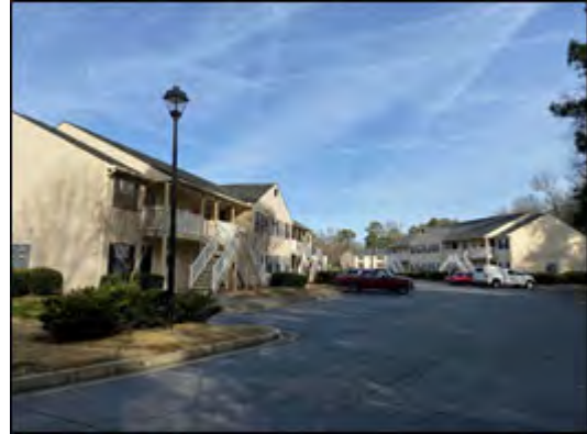
Typical View of Subject Exterior
