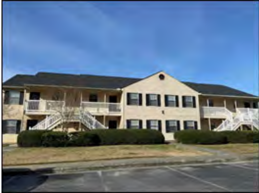
Typical View of Subject Exterior
