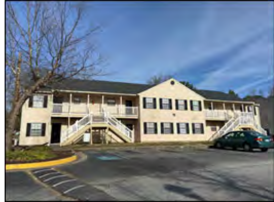
Typical View of Subject Exterior
