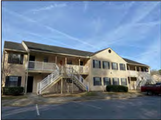
Typical View of Subject Exterior
