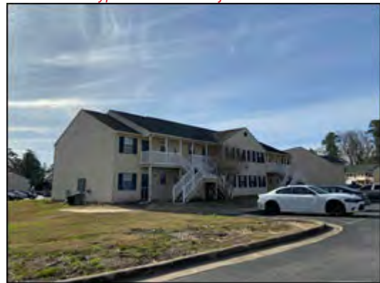
Typical View of Subject Exterior
