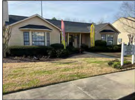
Typical View of Subject Office
