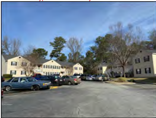
Typical View of Subject Exterior
