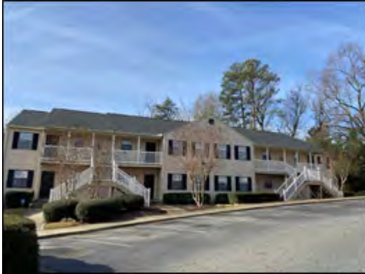
Typical View of Subject Exterior
